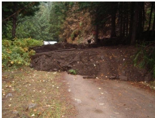
Photo 7 N Ent 2 part of debris flow deposit
