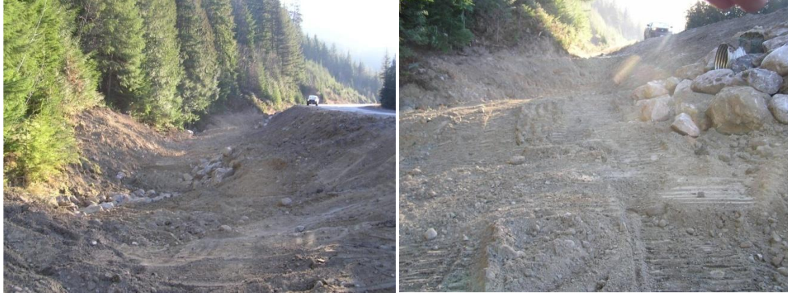
Photos 13 and 14 Additional debris flow storage volume and new overflow culvert installation above highway near middle Van Tuyl Creek
